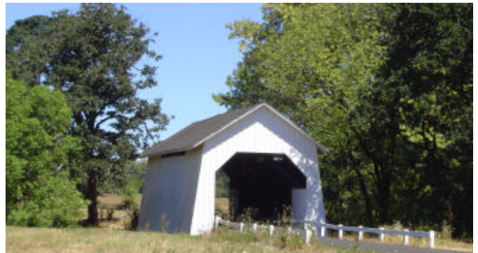
Irish Bend Bridge, Benton County Photo taken by ABHA Staff
